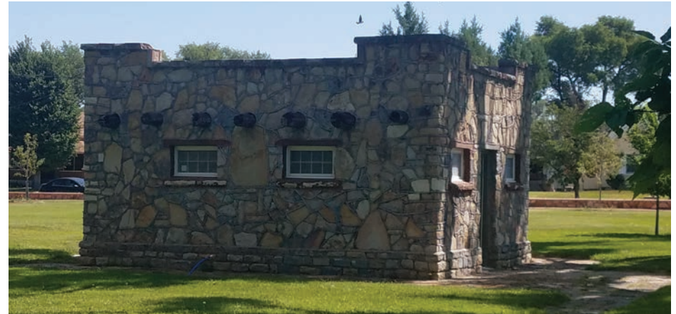
Figure 12: Historic stone structure in City Park is being renovated for public use.
